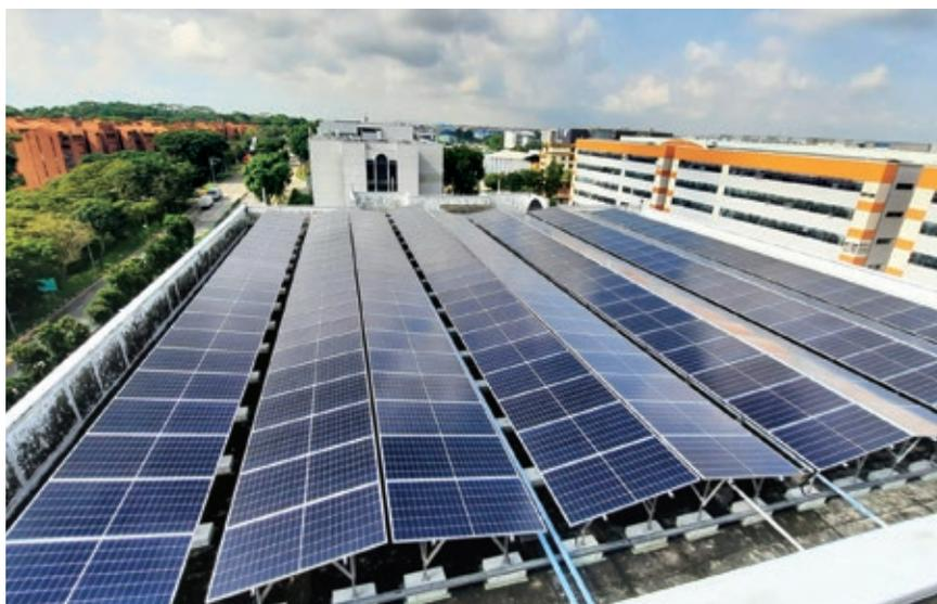
MIT completed the installation of solar panels at five property clusters with an aggregate solar generating capacity of approximately 4,000 kilowatt peak.
